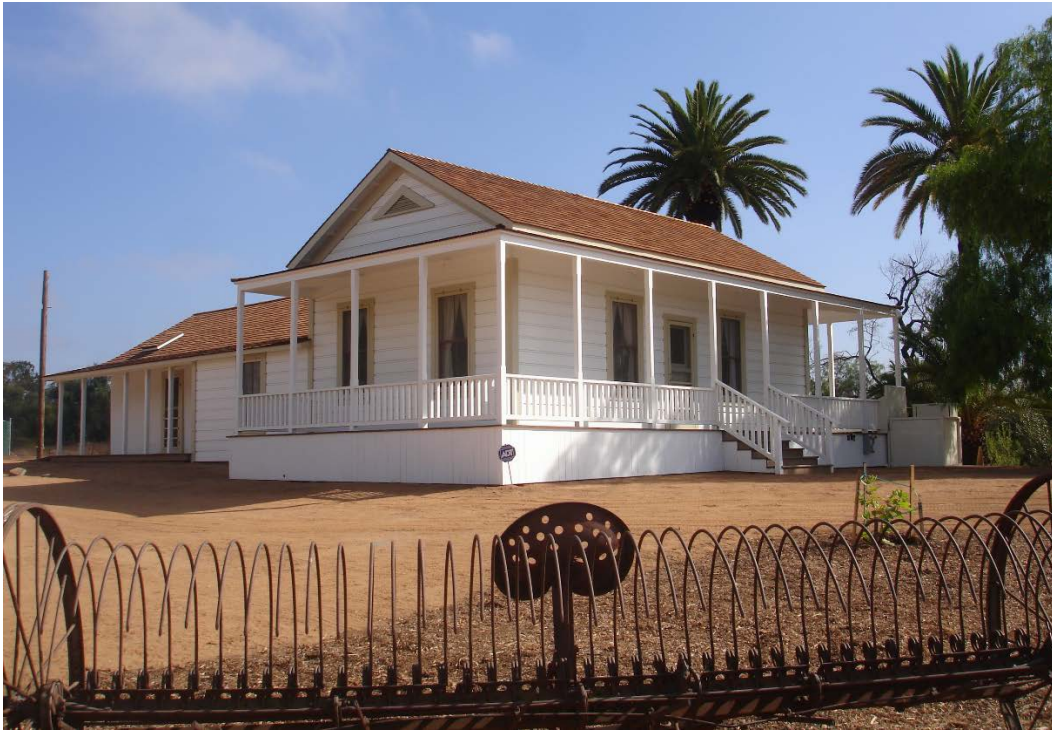
The Sikes Adobe Farmhouse, fully restored to its 1881 period of significance.
