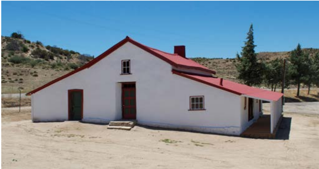
The restored Warner-Carrillo Ranch House and Barn.
