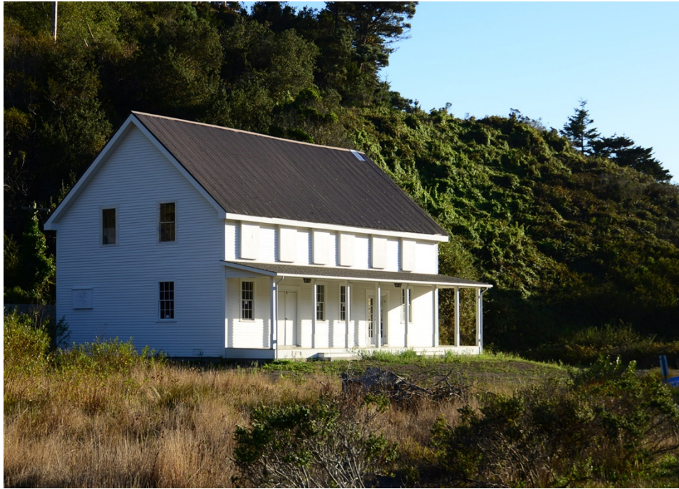
Captain Fletcher's Inn after stabilization and restoration
