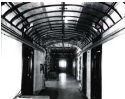
FIGURE 3 Before: GSA Building corridor ductwork installation in progress, 1935.
