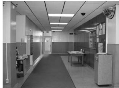
FIGURES 1-2 Thoughtful routing, configuration and concealment of ductwork plays a major role in the esthetic success of HVAC retrofitting projects at historic buildings.
