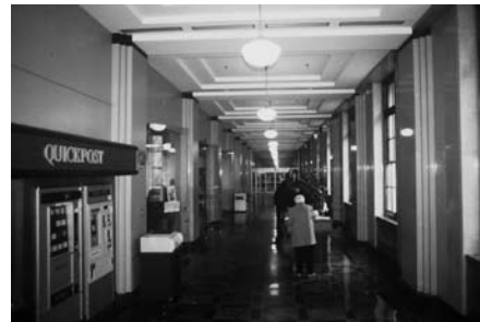
FIGURE 8 Ducts aligned with pilasters and flattened to read as shallow beams blend into historic ceilings.
