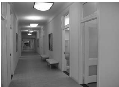
FIGURE 4 After: Relocating corridor ductwork to adjoining office spaces enabled GSA to restore previously concealed cove cornices and door transoms that now flood the corridor with welcomed daylight.
