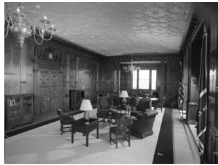
FIGURES 11-12 Linear diffusers located in the plaster walls at each end of this 1917 executive suite increase air supply volume and coverage, reducing the number of wall penetrations otherwise required for conventional grilles. Louvered grilles were confined to end bays and grain painted to blend with the room's paneled oak walls.
