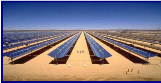
Parabolic trough solar thermal technology
