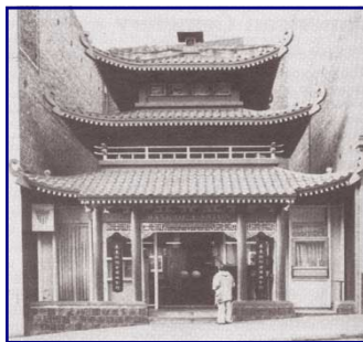
Chinese American Telephone Exchange, San Francisco ( Five Views , p. 148)
