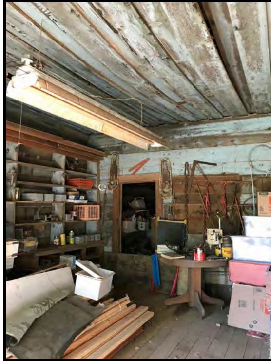
Photo 7. Interior view, Mountain House Historic District, Grocery Store/Post Office, looking northeast (Photo by Corri Jimenez).
