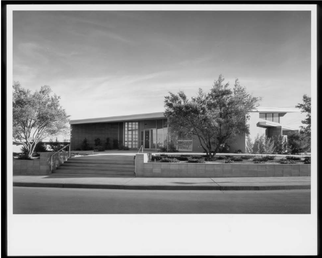
Figure 2. Primary (north) and west elevations, looking southeast 1959.
