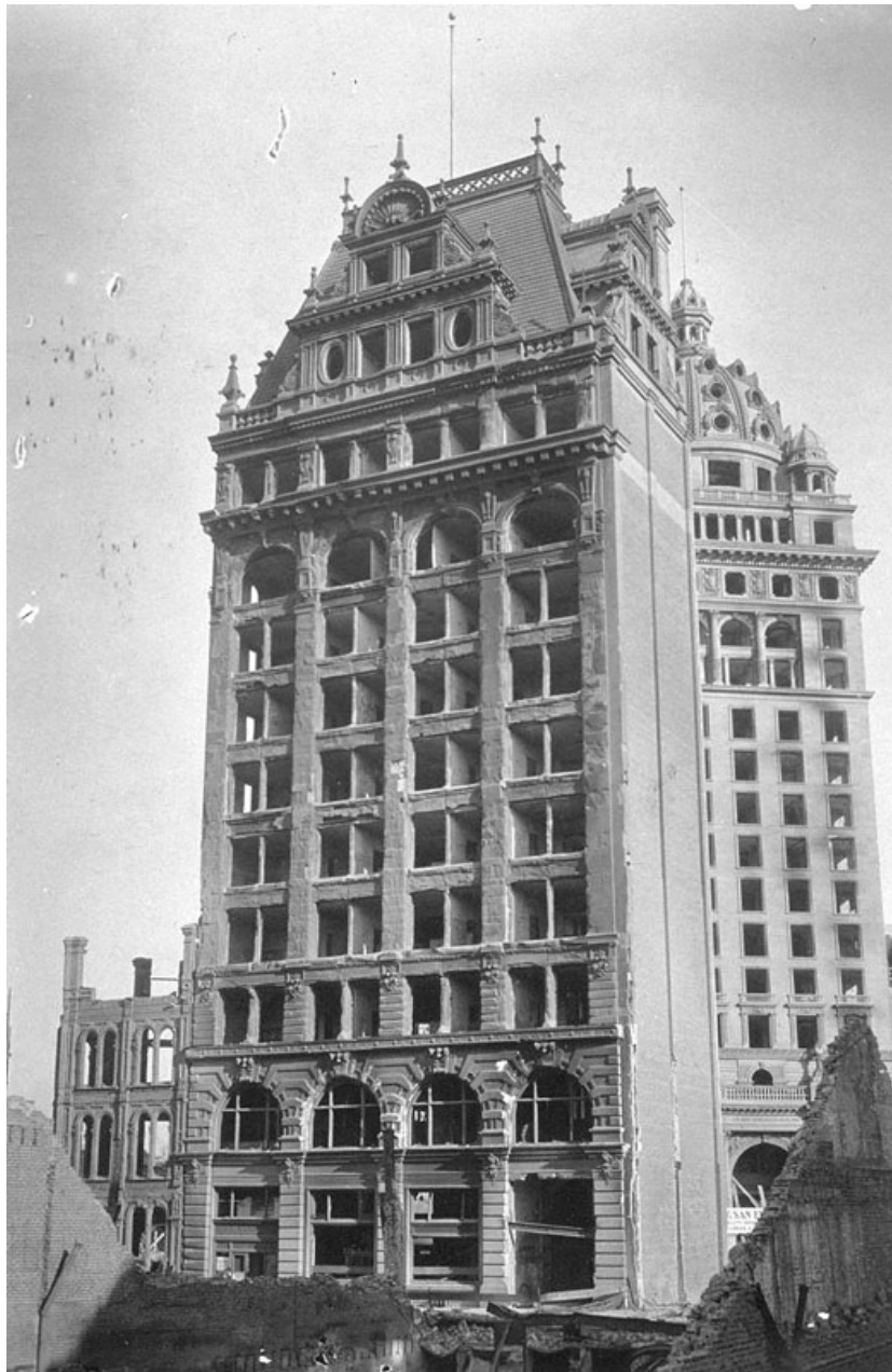
Figure 2: 1906 image of Mutual Savings Bank Building after Earthquake and Fire, view from northwest (image courtesy of UC Berkeley, Bancroft Library).
