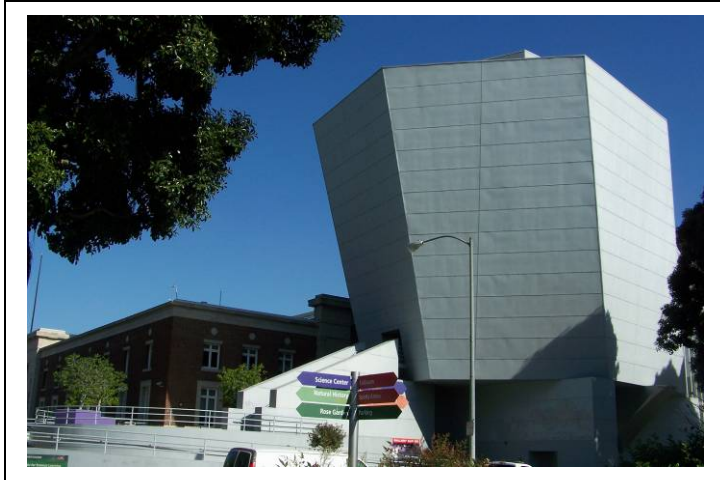
Photo 07: West elevation looking northeast
