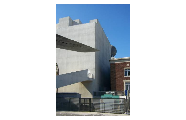
Photo 14: East and north elevations looking southwest
