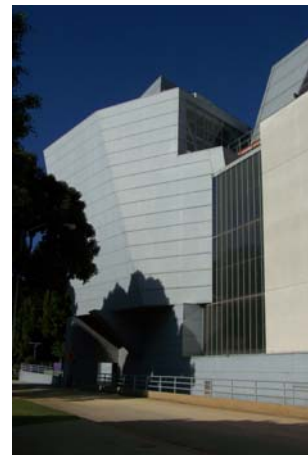
Photo 16: South elevation, looking northwest
