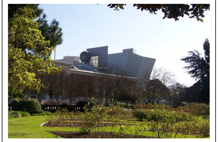
Photo 02: North elevation and armory from across Rose Garden looking southeast
