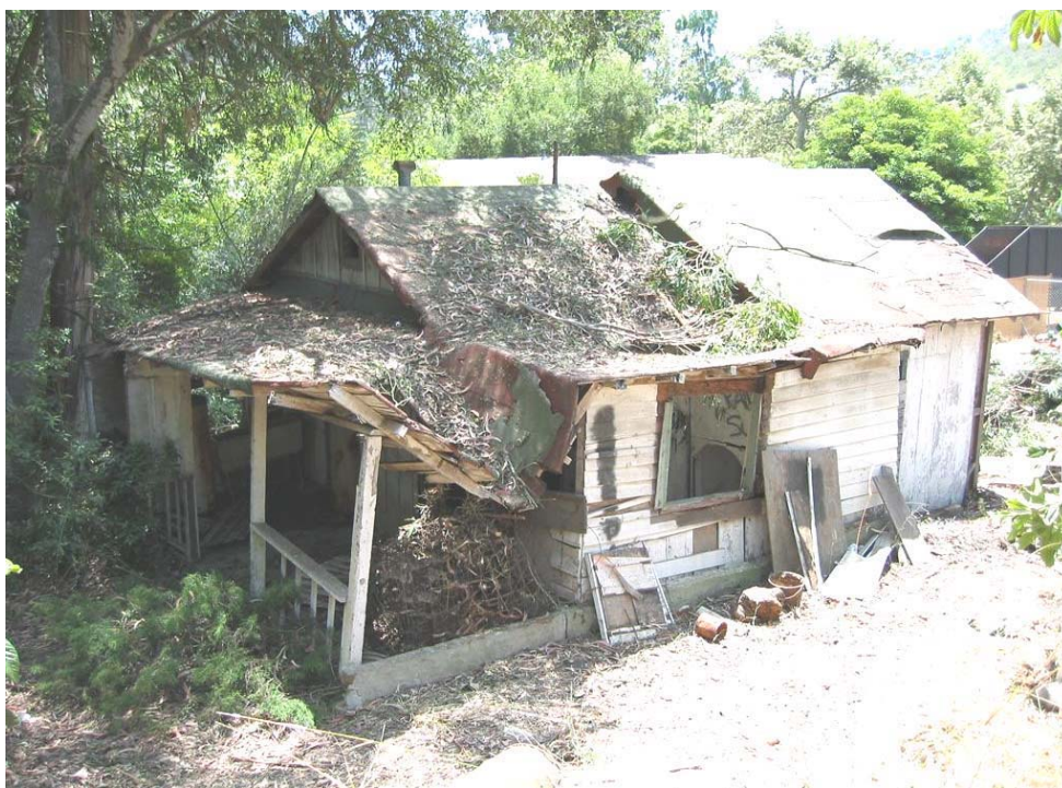
Plate 5. North and east elevations of cabin before porches were removed for repair. Facing south west. 2002. Courtesy Linda Dye
