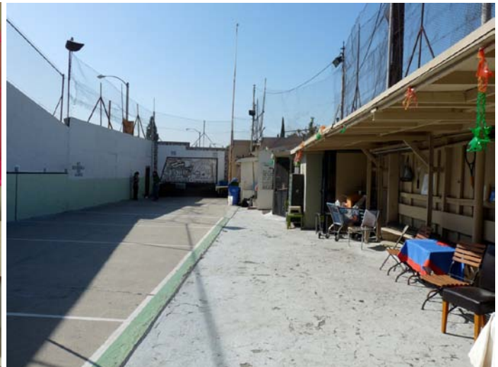
West wall of Maravilla Handball Court, view looking south.
