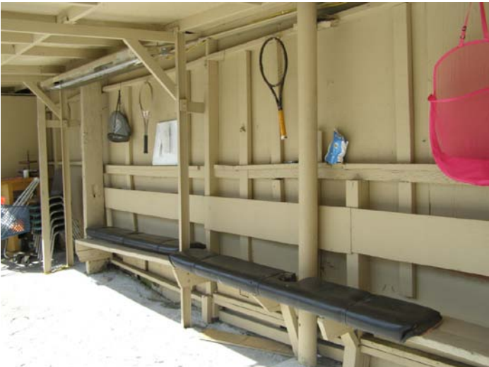
West wall of Maravilla Handball Court, note built-in benches.
