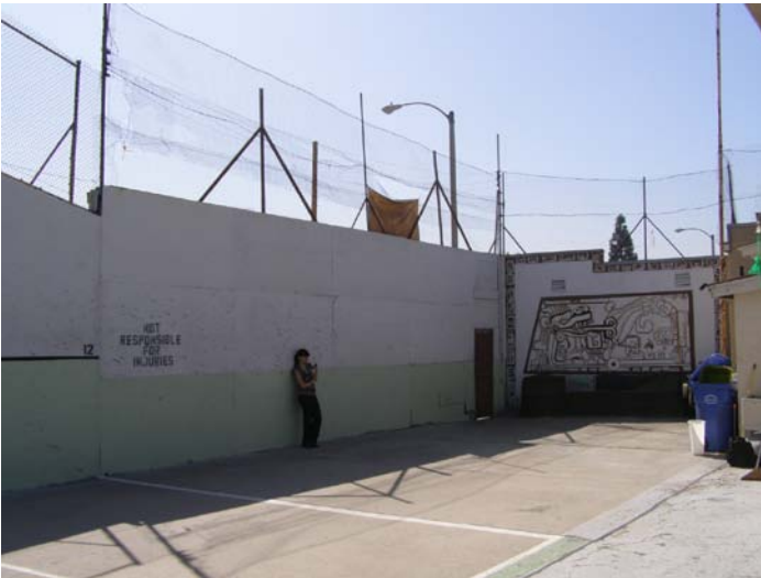
Interior of Maravilla Handball Court, view looking south.
