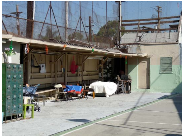
Interior of west wall and storage building at northwest corner of handball court.
