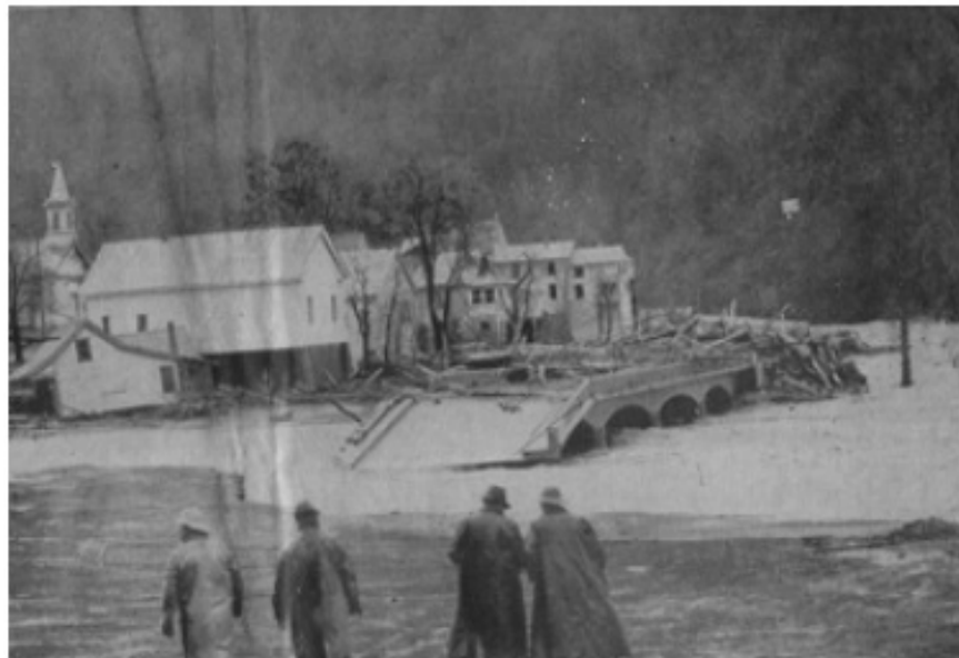
Figure 3. Historic photo of damaged highway bridge, 1937
