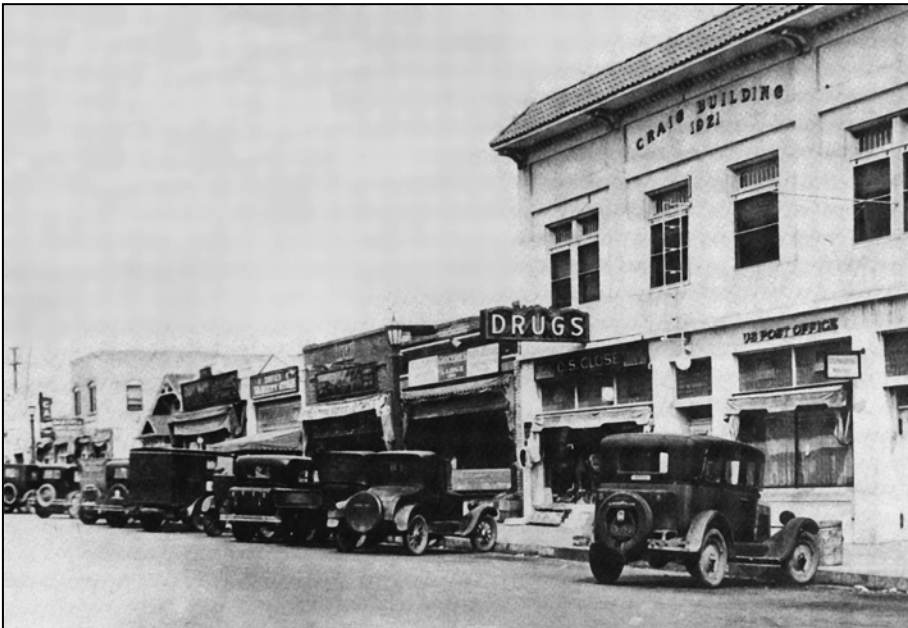
The Craig building, completed in 1921, housed many important functions upstairs on the second floor. Brea's post office and drugstore occupied the first floor. The building was located on the east side of Pomona Avenue (Brea Boulevard) just north of Birch Street.
