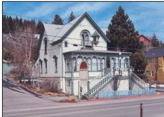
Kruger House/CB White House
