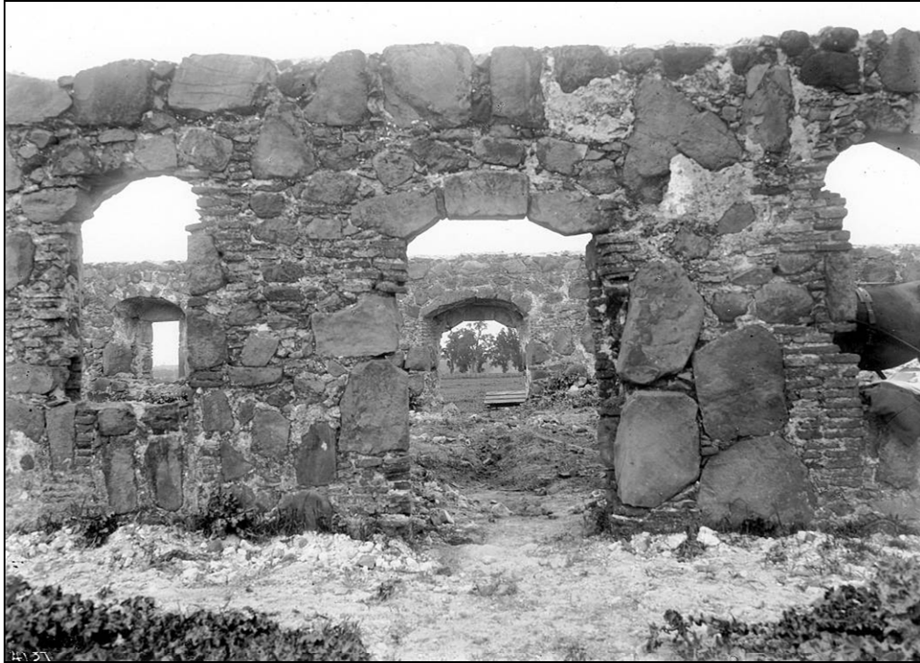
Figure 4-4 South wall of the asistencia, circa 1900 (courtesy University of Southern California, on behalf of the USC Specialized Libraries and Archival Collections).
