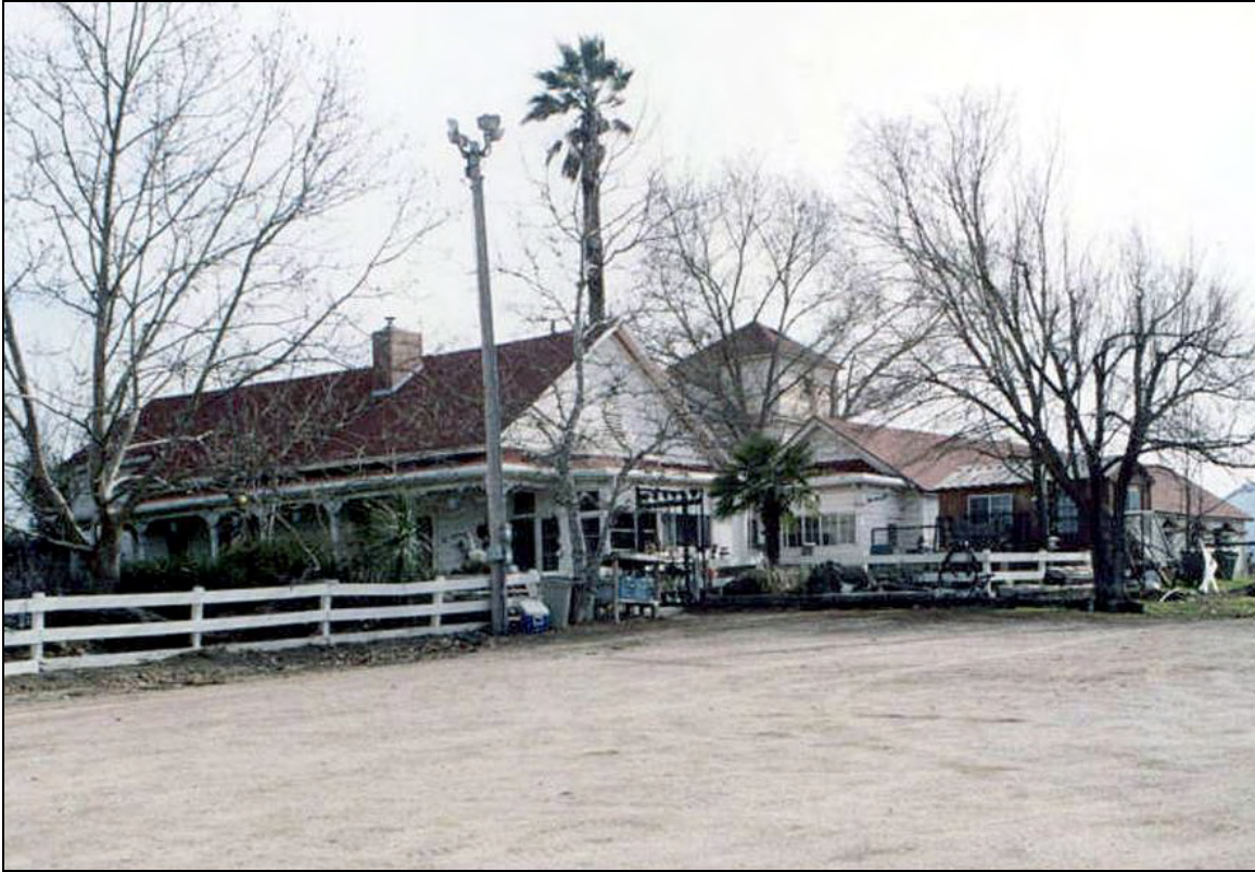
Figure 4-11 Ranch house, facing southeast.
