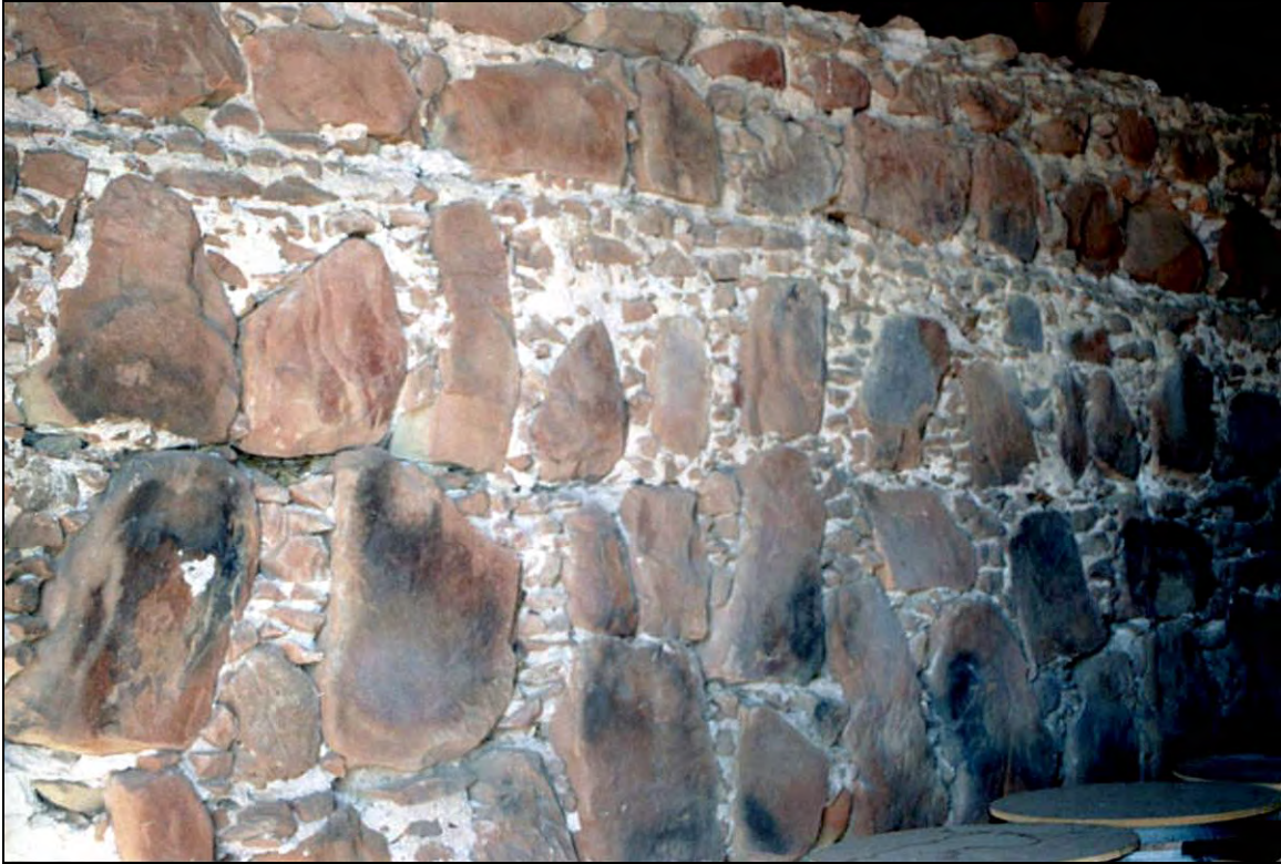
Figure 4-2 Interior north wall of the main asistencia building, facing northeast.
