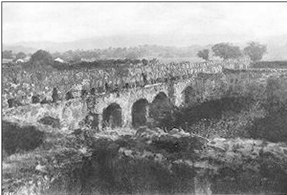
Figure 4-8 Photograph of interior walls of the asistencia, circa 1900 (courtesy University of Southern California, on behalf of the USC Specialized Libraries and Archival Collections).
