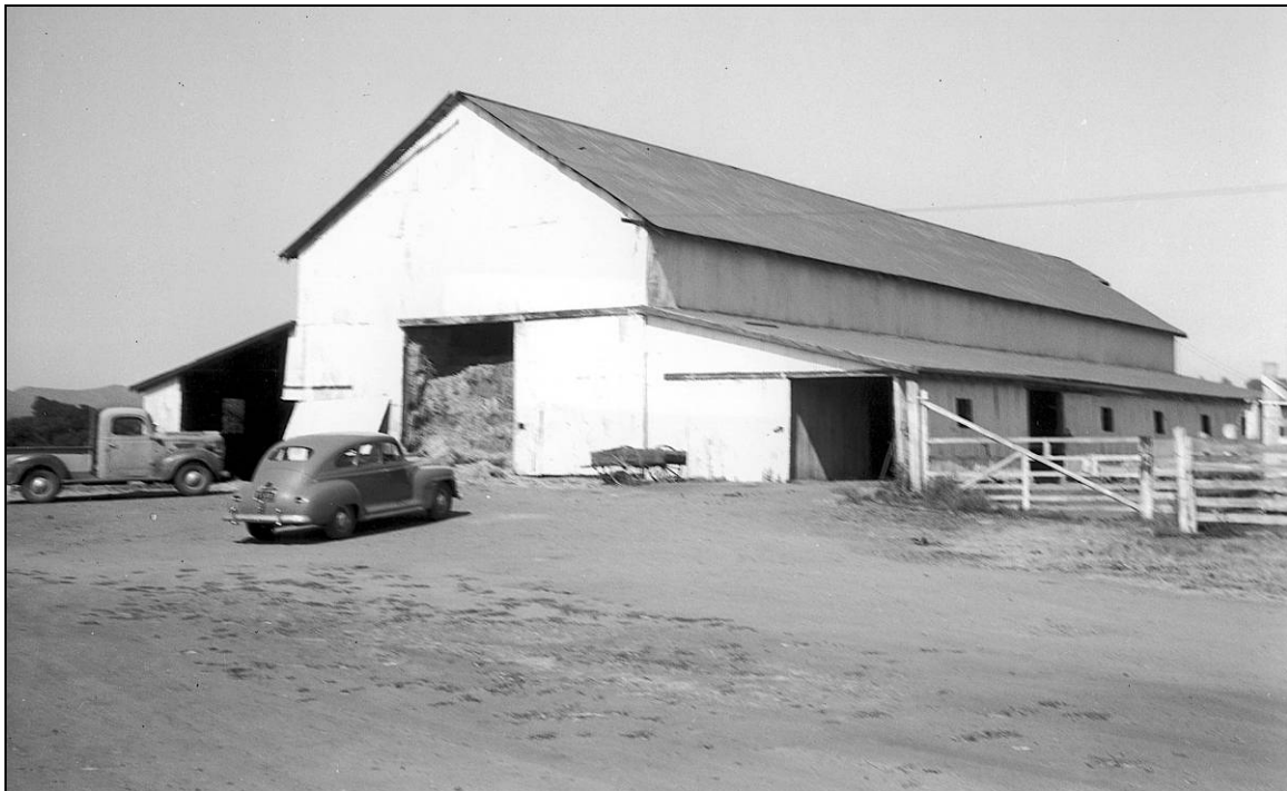
Figure 3-6 The main asistencia building as hay barn, 1951 (reproduced by permission of The Huntington Library).
