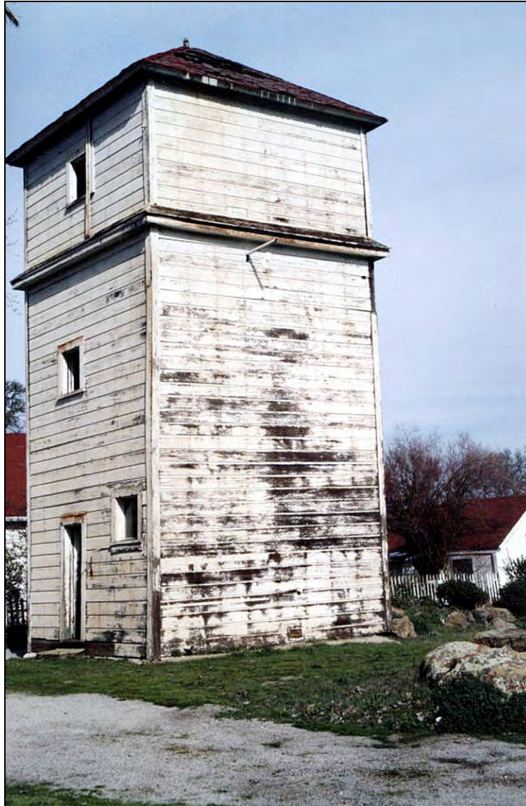
Figure 4-12 Tank house, facing northeast.
