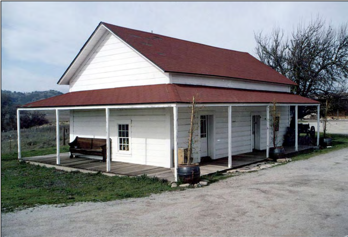
Figure 4-13 Wells Fargo building, also called the Alhambra and stage stop, facing northwest.
