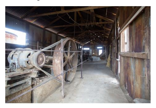
**Photo 14** General view of the building's interior and almost the whole operating system, including a top view of electric motor and v-belts on the drive wheel, the long drive belt on the left of the photo, and machinery at the far end of the Jack Plant. The camera is facing south.
