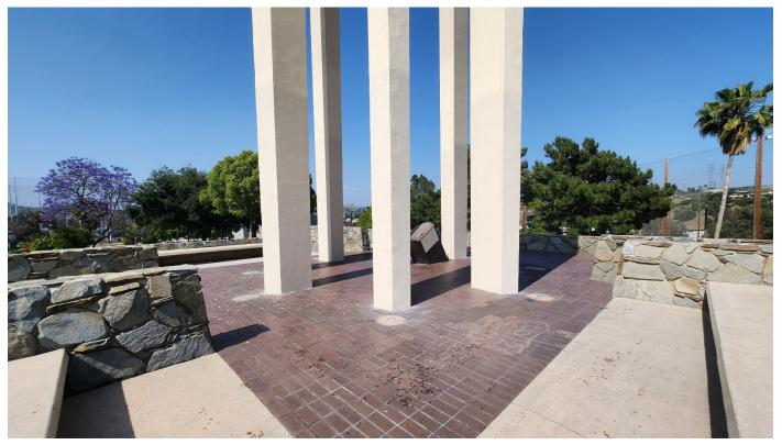
Photo 10. Detail view of monument base with stacked bond brick pavers and integrated concrete benches; camera facing southwest.
