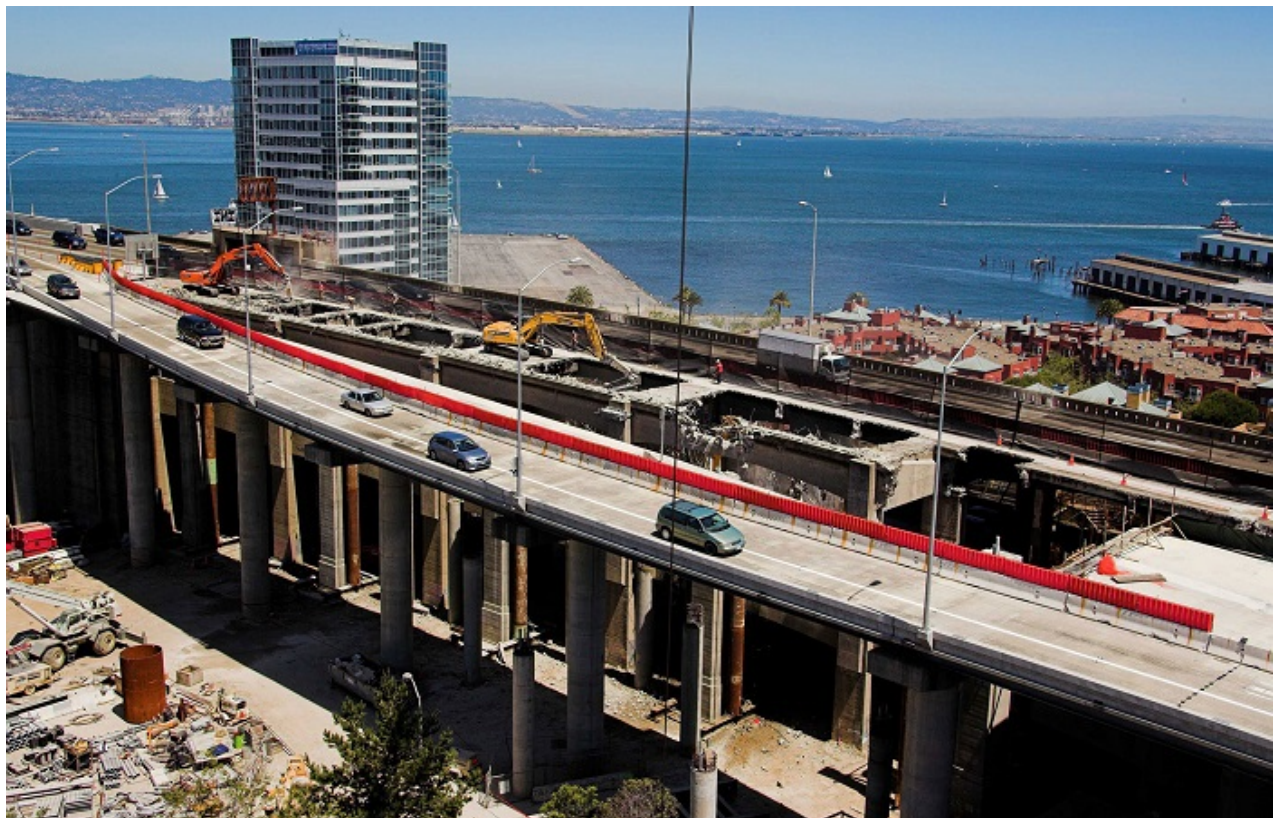
Figure 2. Demolition of San Francisco Approach. Undated Caltrans photo,
