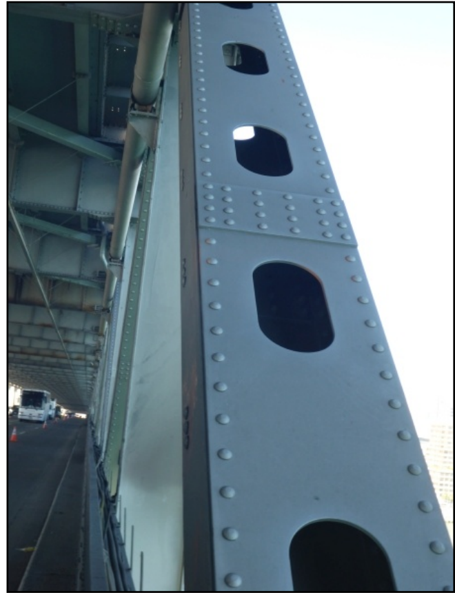
Figure 4: Northern truss member, Span W2, PP84, Lane 1, taken 7/20/17.
