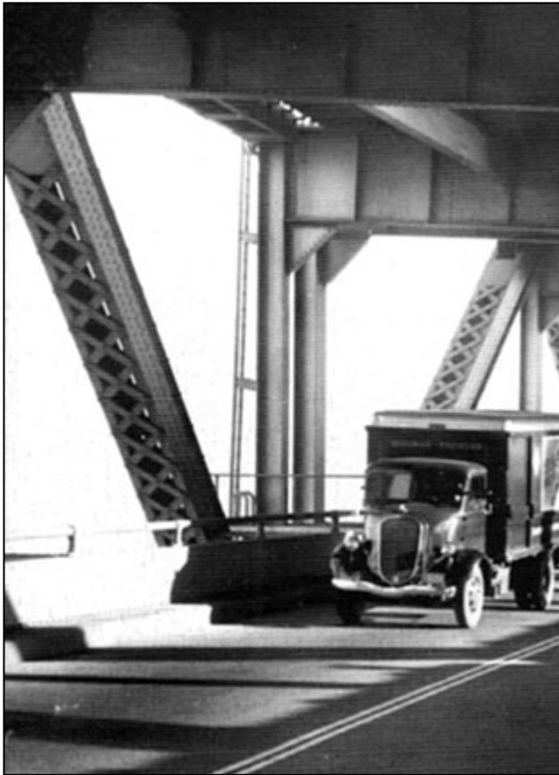
Figure 3: Lower deck, showing lattice truss members, image from "Bay Bridge Artery," Chris Carlsson, 2013, www.foundsf.org , accessed 1/24/20.
