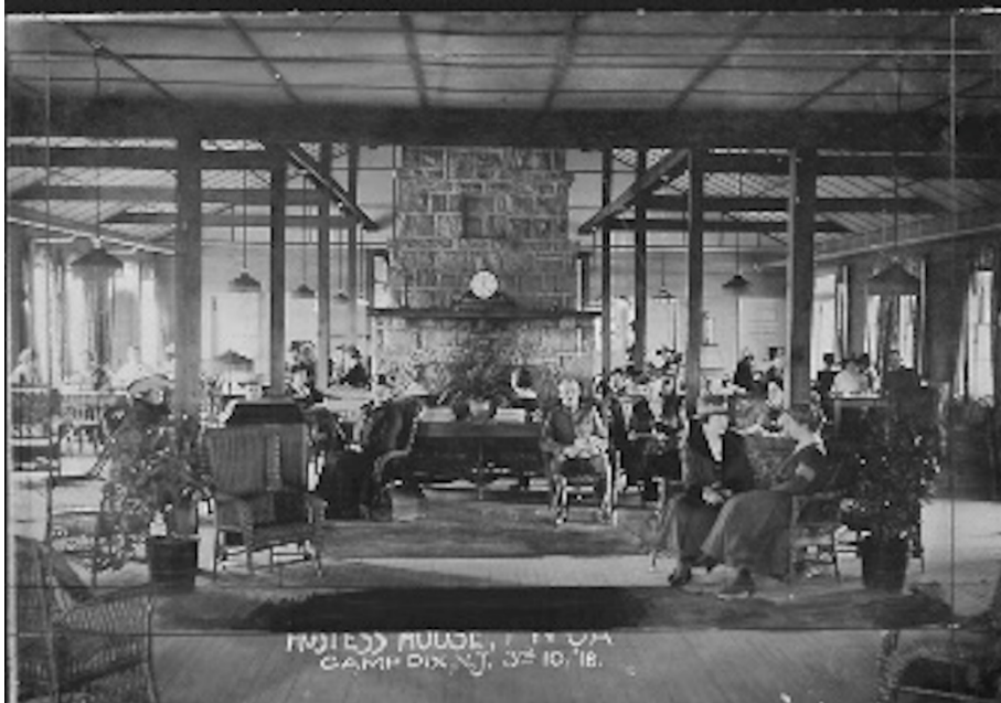
Figure 3 Hostess House Camp Dix, New Jersey with two separate buildings for black and white servicemen—note large brick or stone fireplaces with decorative elements, large windows, encased beams and posts, wide porch, inglenook sitting area, shingled exterior siding
