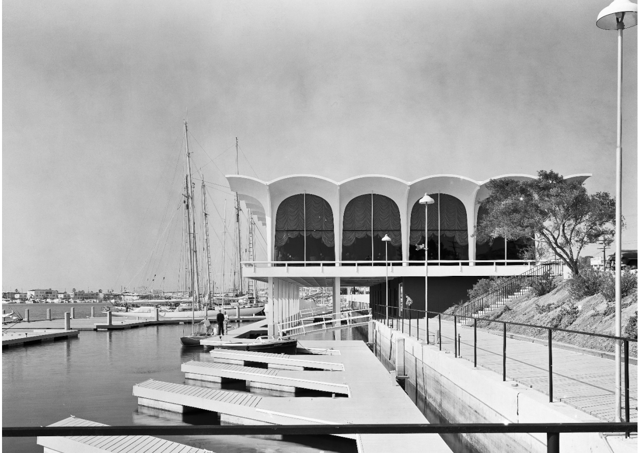
Figure 5. Stuft Shirt restaurant building, view west, 1960, photograph by Ezra Stoller (courtesy © Ezra Stoller/Esto).
