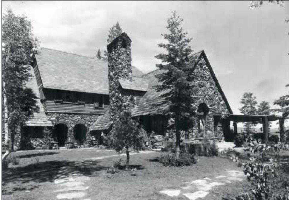
South façade, Westphal Summer Residence.
