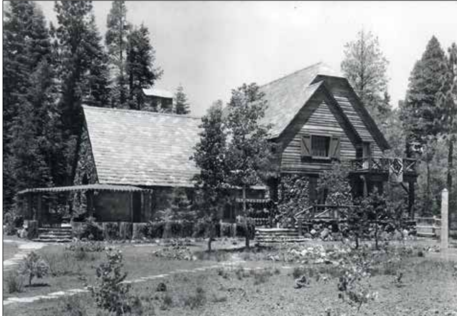
East façade, Westphal Summer Residence.
