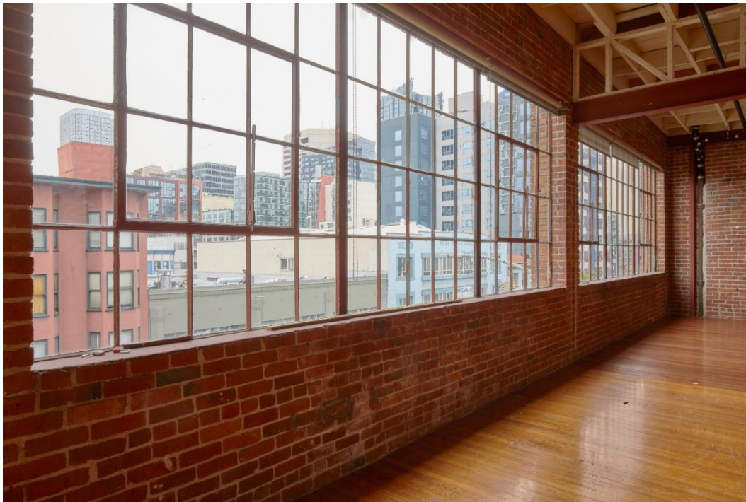
Photo 14 Detail of divided-lite steel window at third story. Looking northwest.
