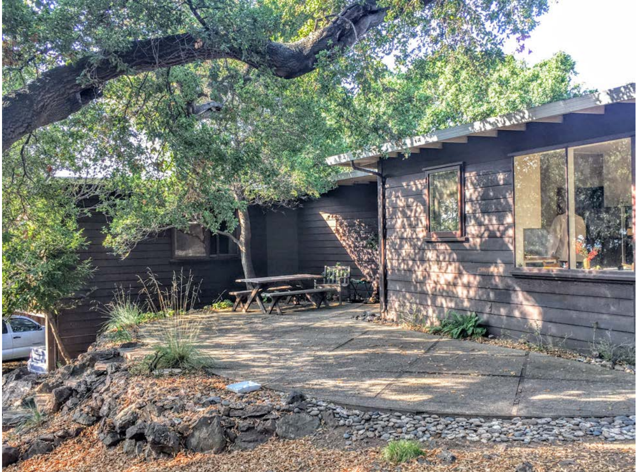
Photo 2 of 10. Front terrace and kitchen, looking SW
