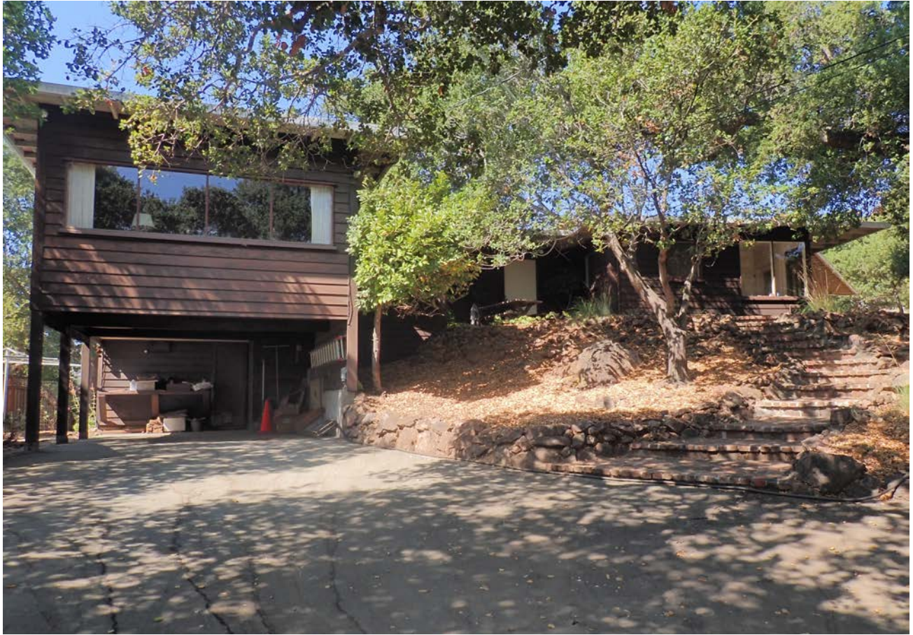
Photo 1 of 10. Front elevation, east side of house
