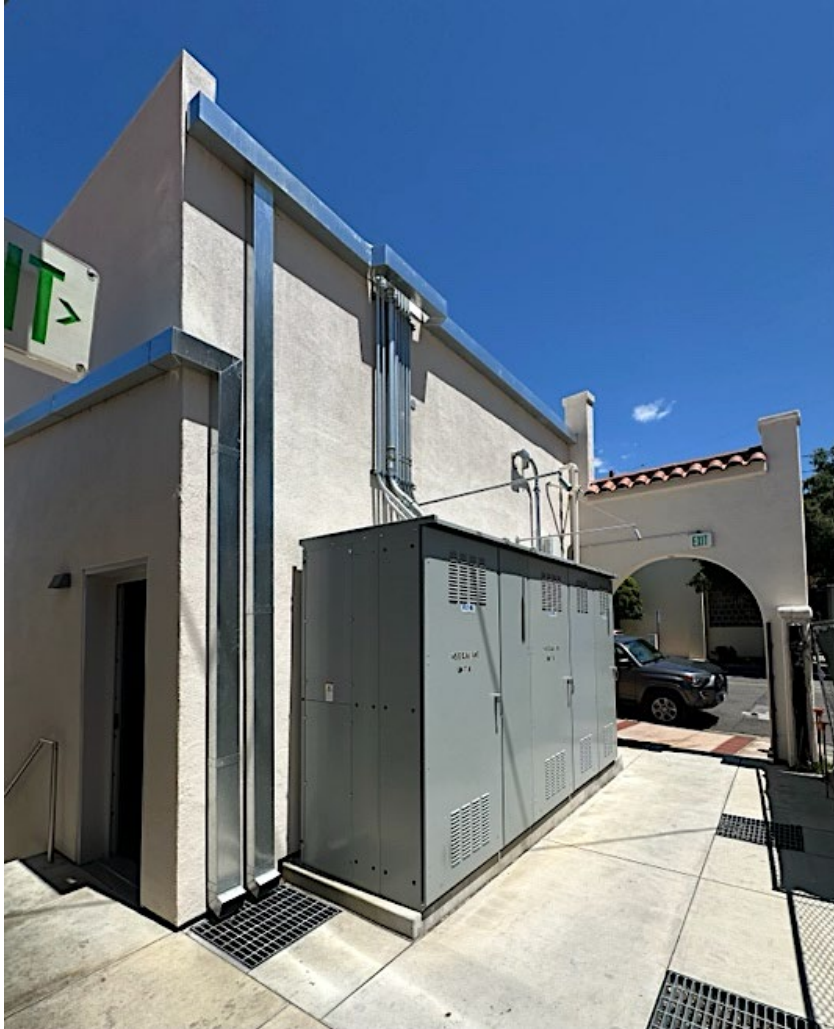
6 of 22 (CA_Ventura_IsisTheater_0006) Rear elevation of theater. View: NE.
