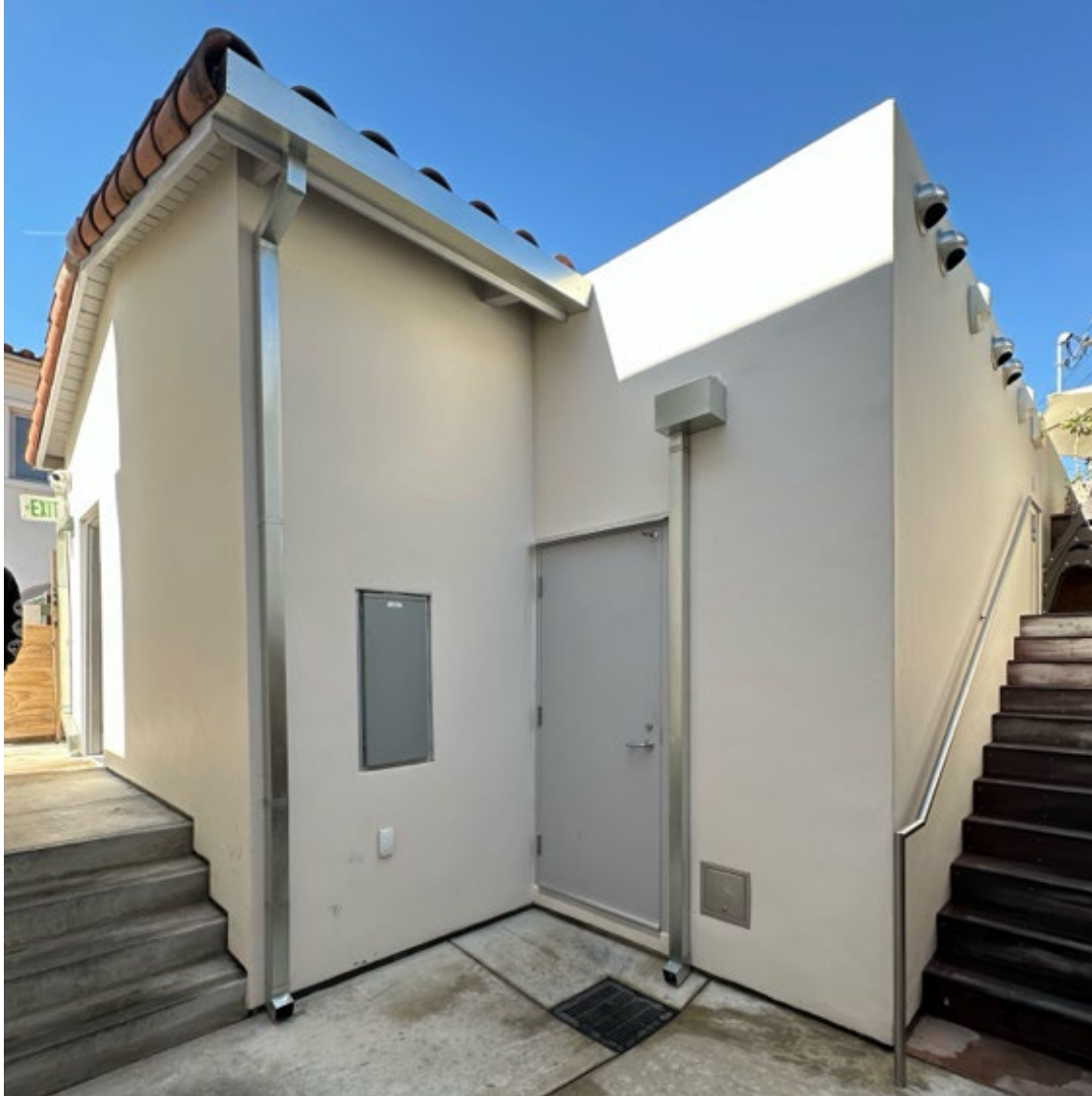
12 of 22 (CA_Ventura_IsisTheater_0012) Former Love's Cleaners, recent addition. View: SW.
