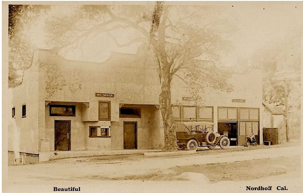
Figure 1. Isis Theater front elevation of 1914-1916. Carole Denardo and Craig Walker. "Final Report: Historic Resource Inventory and Evaluation, Ojai Playhouse Theater, 145 East Ojai Avenue (APN 023-0-077-050), Ojai, Ventura County, California." technical report (Santa Ynez, CA: Provenience Group, Inc., July 22, 2019), cover.
