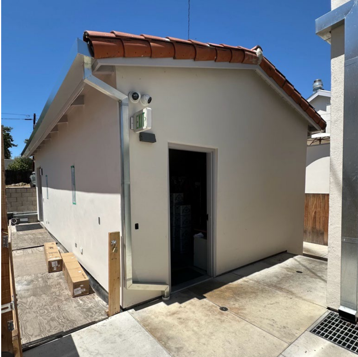
11 of 22 (CA_Ventura_IsisTheater_0011) Former Love's Cleaners, front and side elevation. View: NW.
