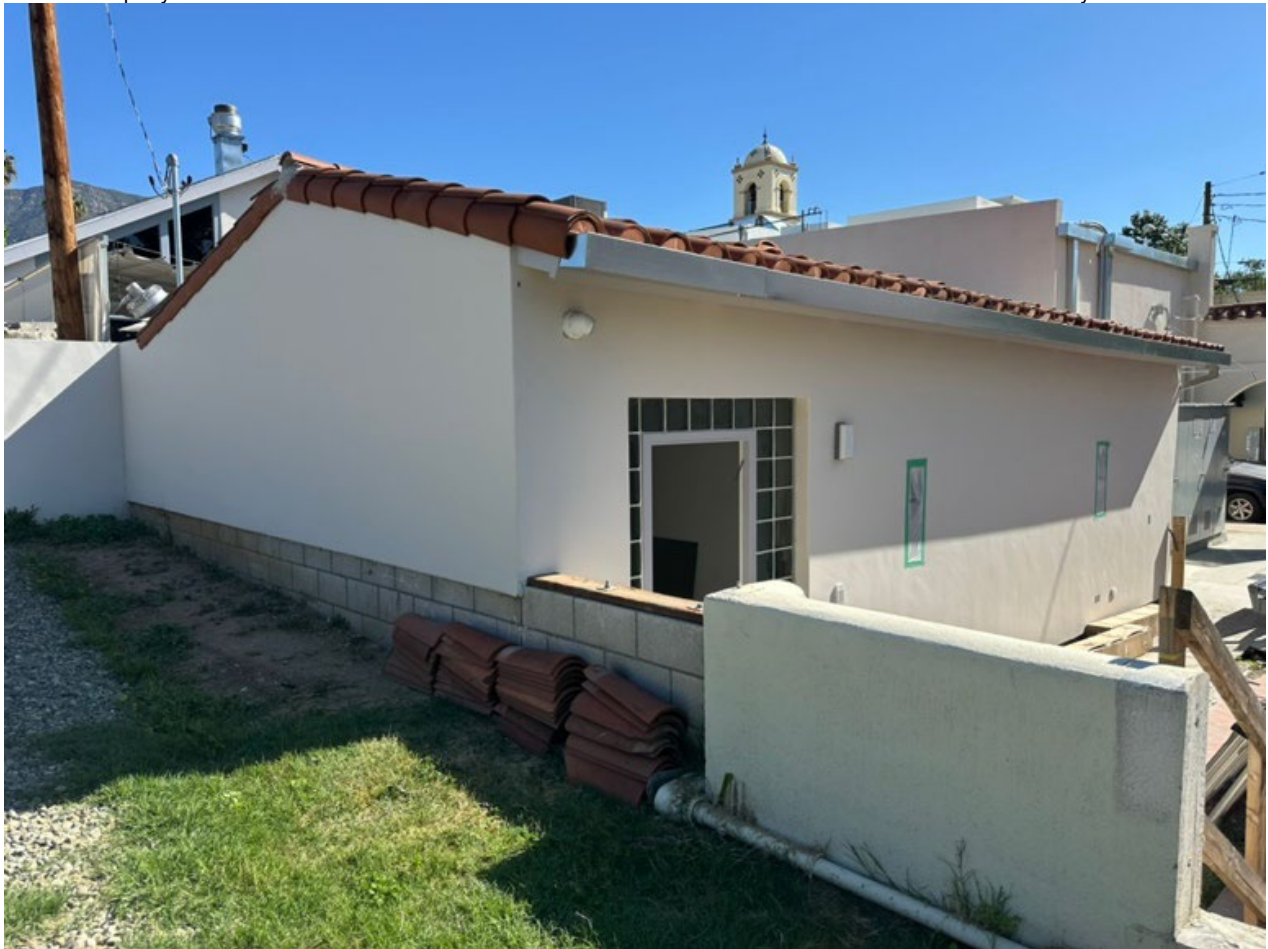
9 of 22 (CA_Ventura_IsisTheater_0009) Former Love's Cleaners at SW portion of parcel. View: NE.
