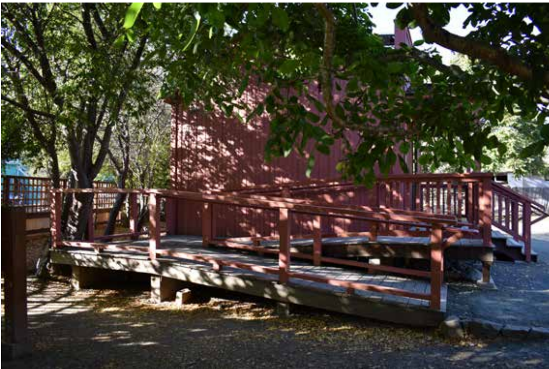
Secondary (South) Elevation of Cambria Chinese Temple North-Facing View; Photo Taken 10/28/2019
