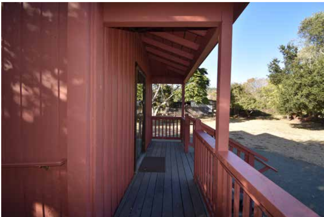
Porch of Cambria Chinese Temple North-Facing View; Photo Taken 10/18/2019
