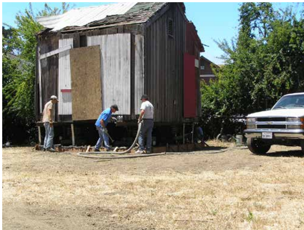
Cambria Chinese Temple Following its Relocation, Prior to its Placement on New Foundation Photo Taken July 6, 2007
