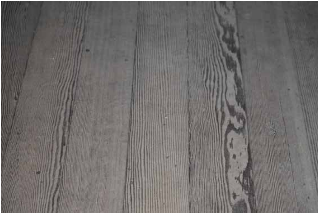
Close-up of Floorboards on Interior of Cambria Chinese Temple Photo Taken 10/18/2019
