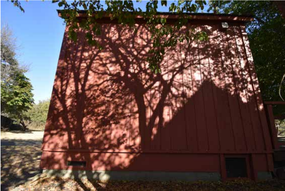
Rear (west) Elevation of Cambria Chinese Temple East-Facing View; Photo Taken 10/28/2019
