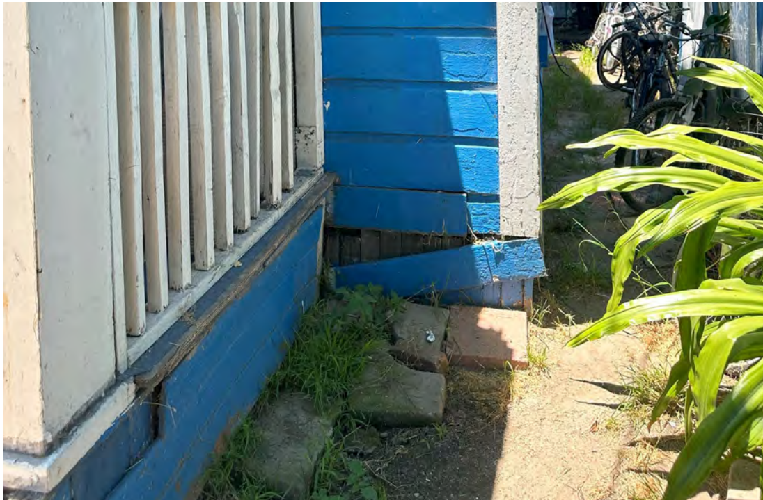
Image 4: Close-up Elevation Exposed Deteriorated Crippler Wall.
