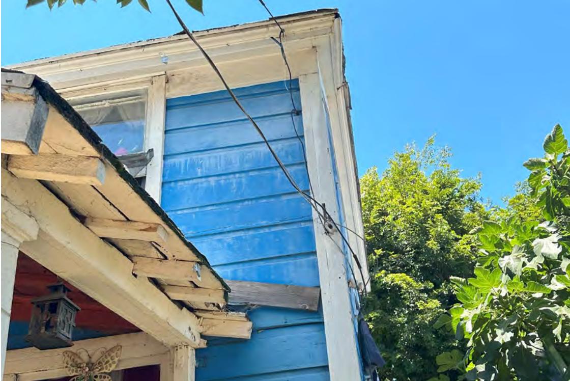
Image 4: East Elevation Close-up Exposed Siding and Damaged Roof Edges.
