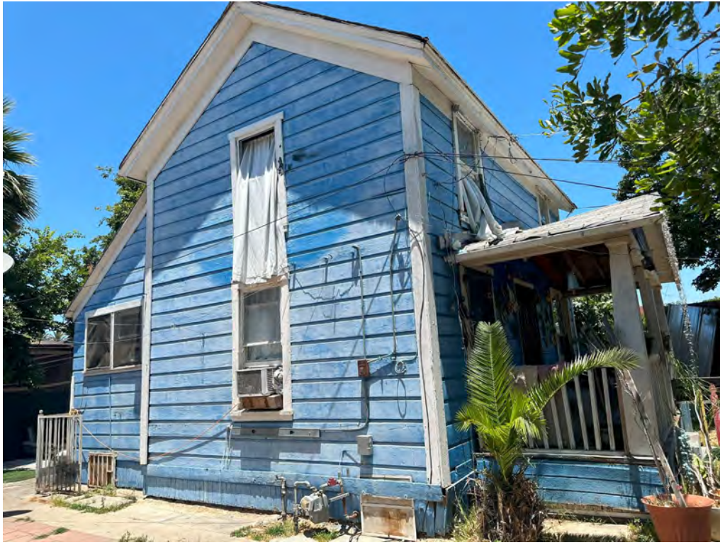
Image 1: South Elevation – Condition of the Roofing and Siding are Beyond Repair. Soft / Nonexistent Backing Observed.
